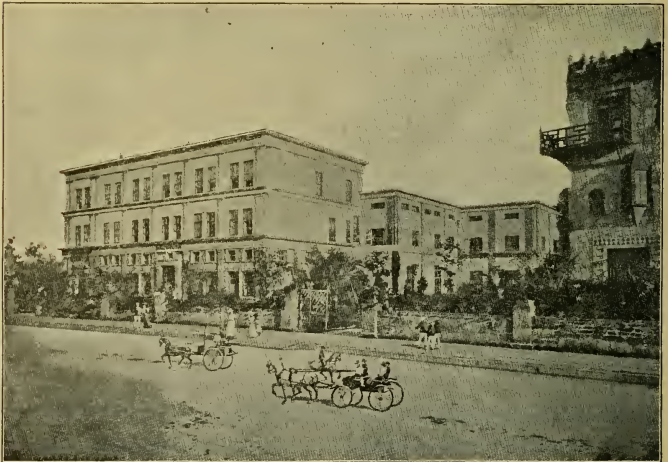
No. 47 is of the Hotel Granada, St. Augustine. The first story is of solid concrete. The second and third stories are of concrete in metal lathing \frac{3}{4} inch in thickness.
