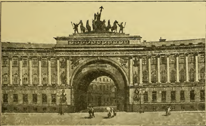
No. 126.—Portal through the War Department buildings, St. Petersburg.
