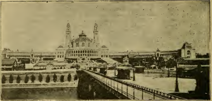
No. 14.—Exterior of the Trocadero Galleries, Paris.
