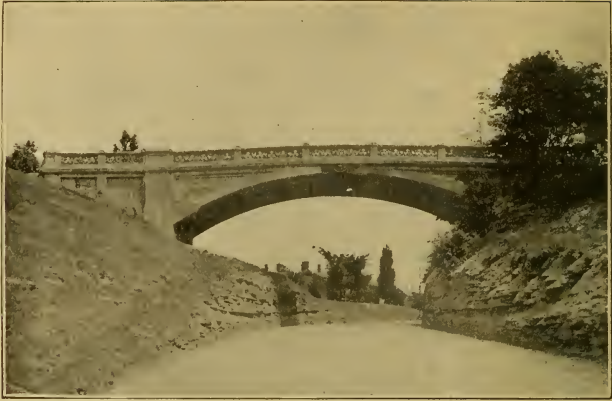
No. 130.—Melan arch-bridge construction, Eden Park, Cincinnati.
