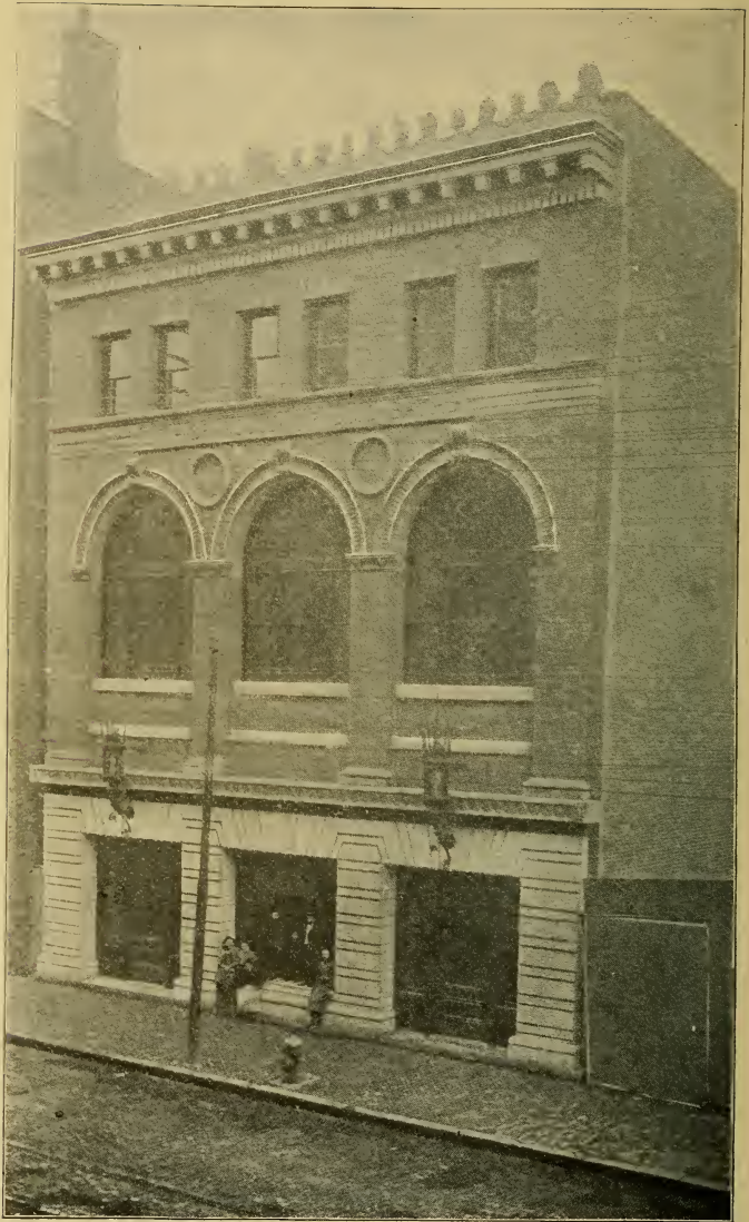
No. 118.—New municipal bath, Dover street, Boston.
